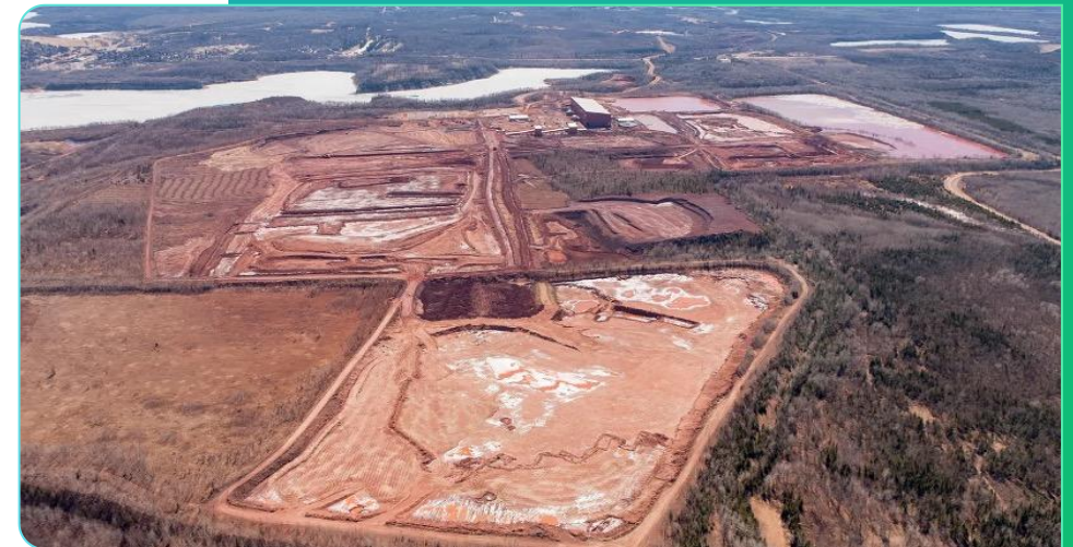
Plant 4 Overhead Photo
